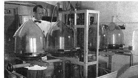
CHARACTRON CATHODE RAY TUBE has vacuum of 2x10 -6 microns. That is one reason the 19-in. tube costs so many more times than a TV tube of the same size.
