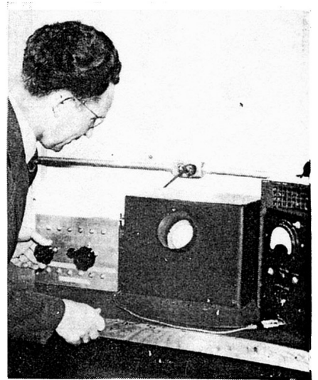
J. T. McNaney of Consolidated Vultee demonstrates his Electrontype system for producing messages or numerical results on screen of Charactron cathode-ray tube in response to coded signals applied to multiple deflecting electrodes
